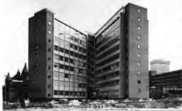
Figure 4 The new hospital in the final stages of construction, Queensway is incomplete.
